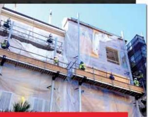
**1500 LB LIFT CAPACITY** The PowerMast is ground supported and has a lift capacity of up to 1500 lbs per twin system.
