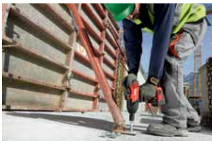
Great for temporary bracing...
