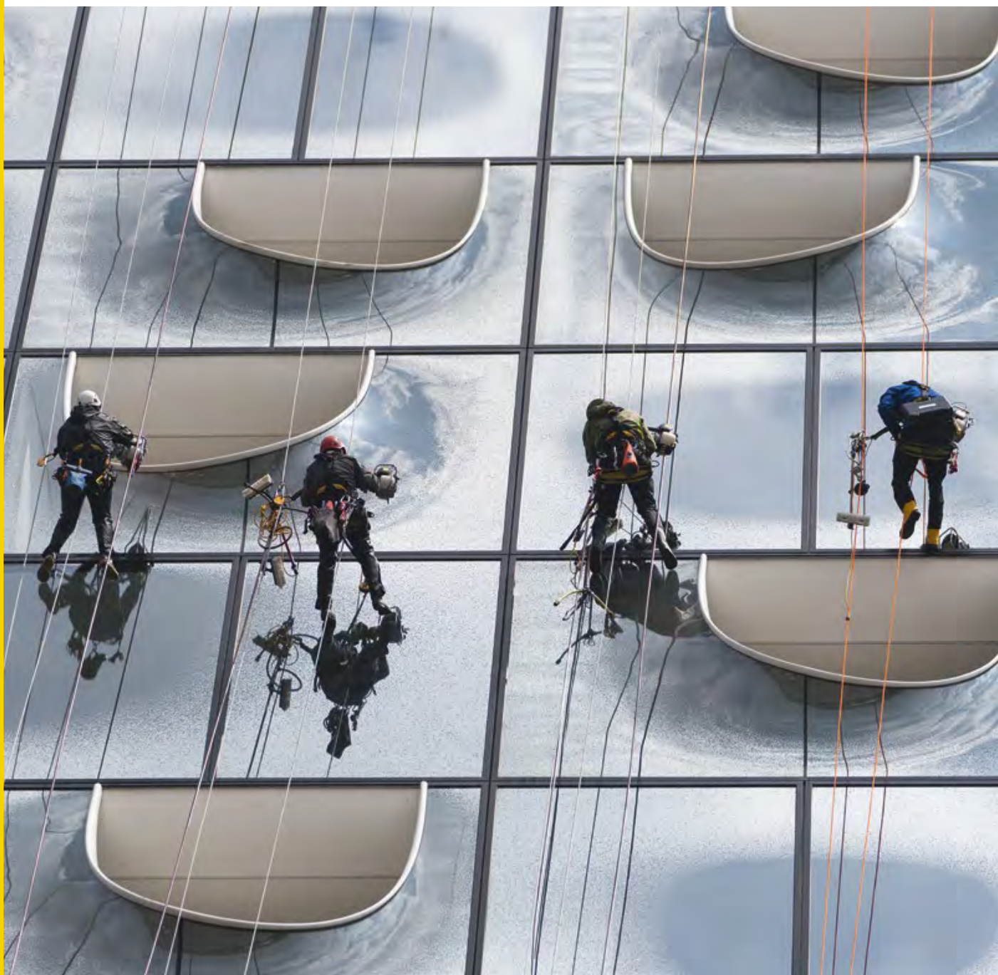
Window cleaning on the Elbphilharmonie building, Hamburg, Germany © Petzl - vuedici.org - 3Ker Ras Group/ABO Glasreinigung - Elbphilharmonie
