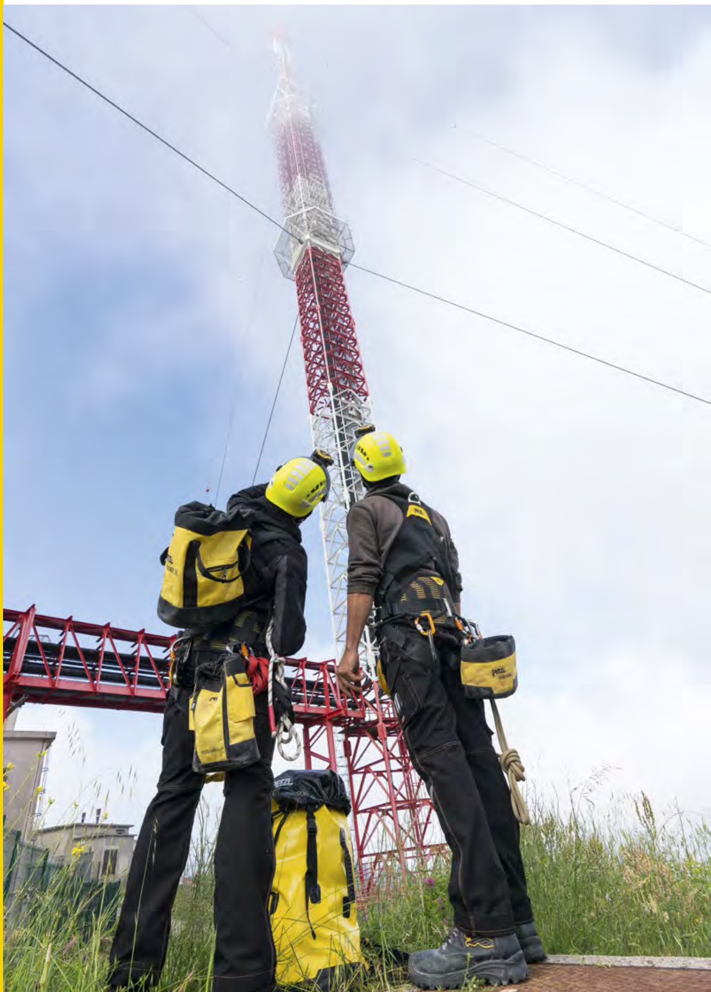
Pylone inspection and maintenance © Petzl - vuedici.org - Profil - TDF
