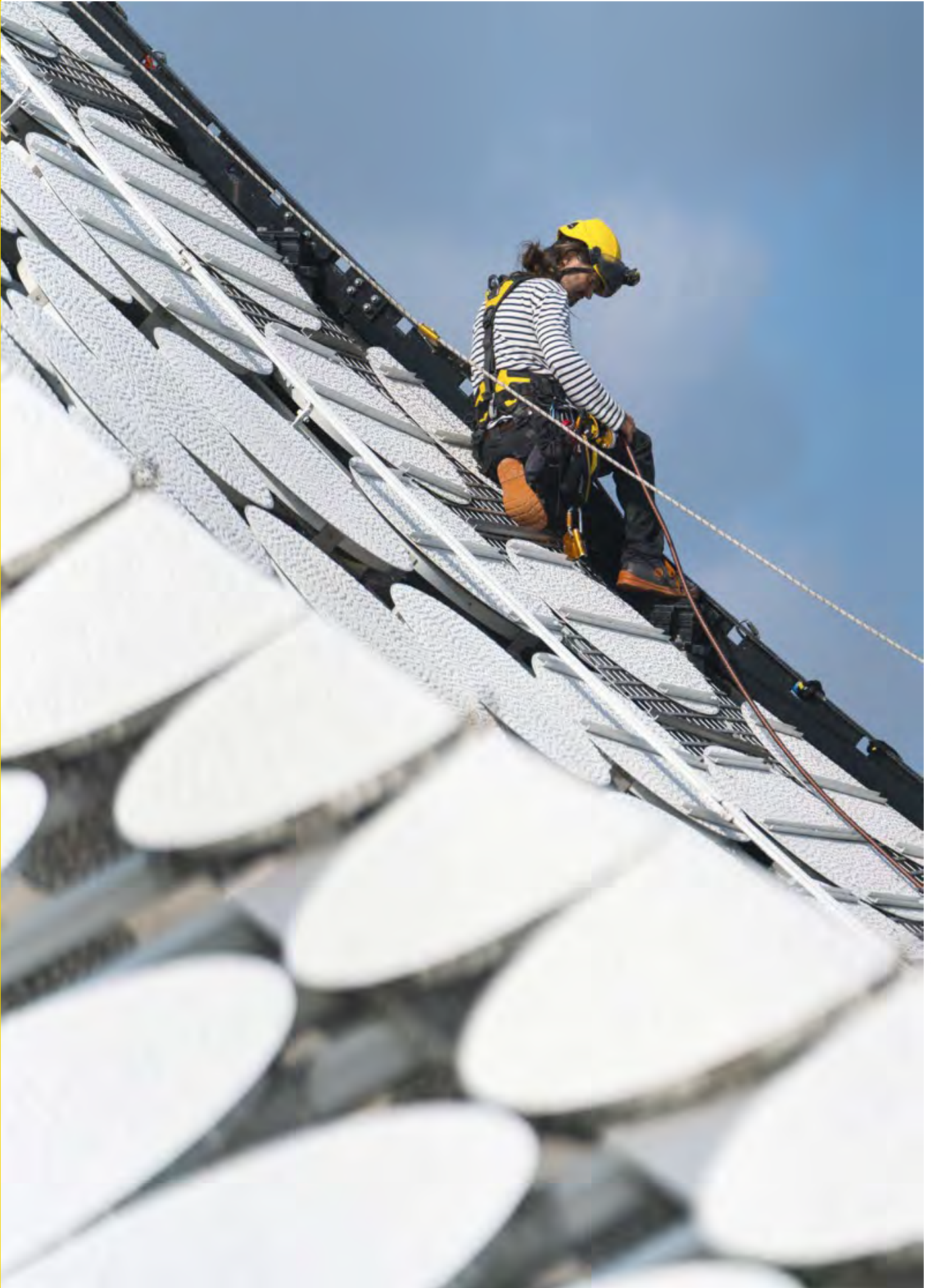
Window cleaning on the Elbphilharmonie building, Hamburg, Germany © Petzl - vuedici.org - 3ker Ras Group/ABO Glasreinigung - Elbphilharmonie
